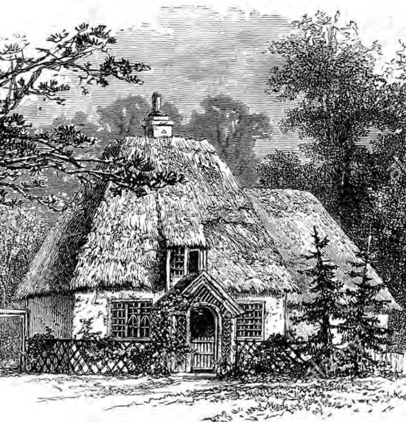
THE DAIRY, ALTHORP.
