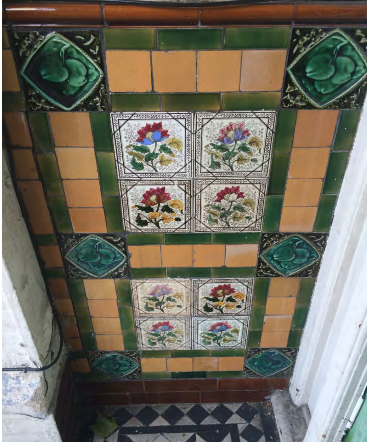
Transfer-printed tiles by the firm Jackson Brothers in the porch of a Victorian house in London, c. 1890
