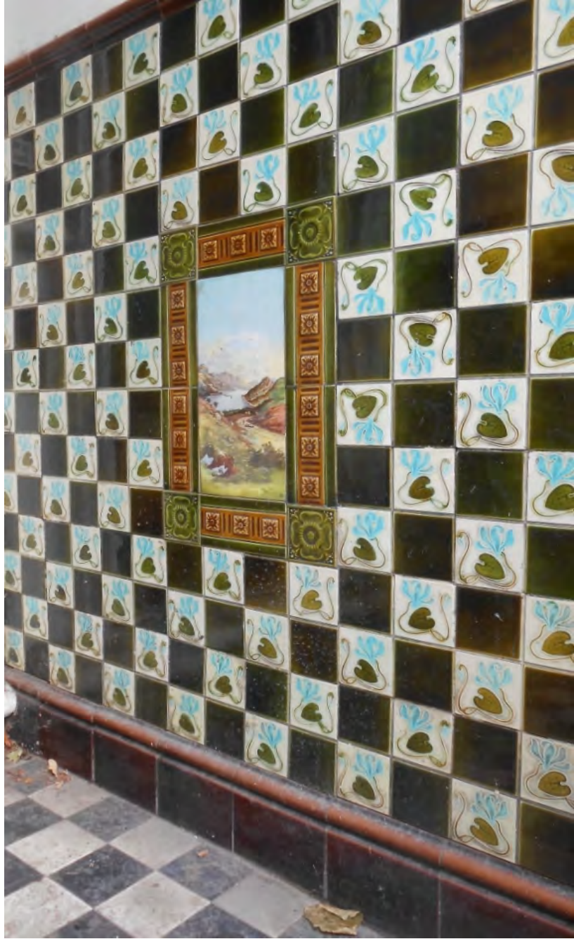
Tiled porch in Hull, c. 1900 -1905
