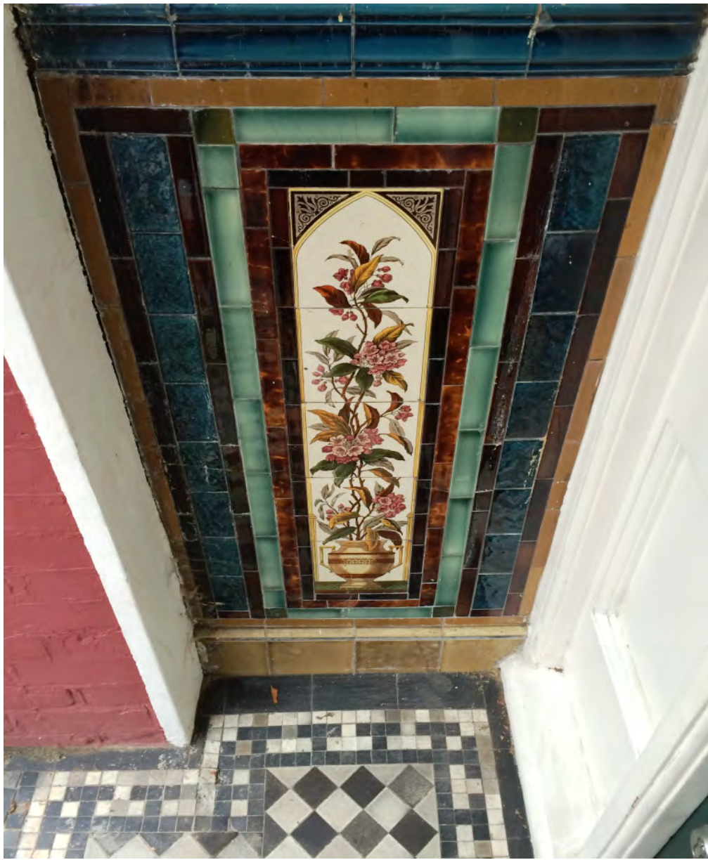
Tiled porch in London with printed tiles by the Decorative Art Tile Co., Hanley, c. 1890
